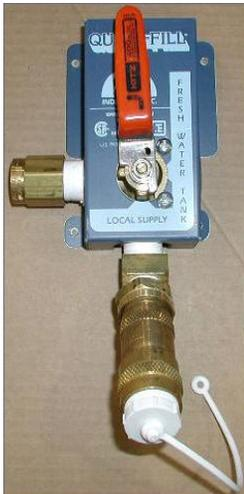
The handle should remain in the local supply position until you are ready to fill the fresh water tank.
