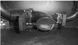
The drainage system, including the tanks and associated drain piping should be periodically inspected for loose fittings from vibrations. Any deterioration of the sealant around joints and fittings should be repaired immediately.
